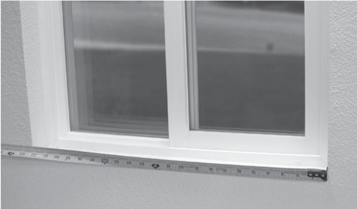
Measure the width of the inside jamb to jamb of the window opening.
