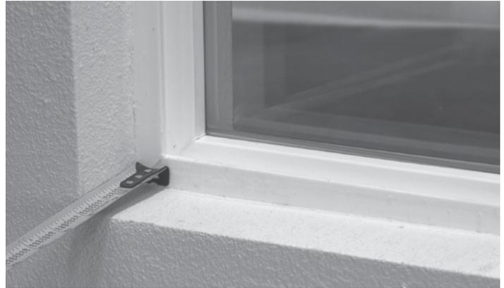
Sill-Rite sills are available in depths from 2 to 8 inches, in one-inch increments, to accommodate different wall thicknesses.
