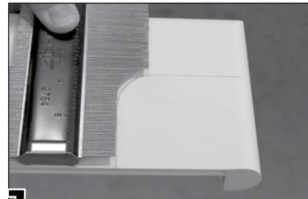
**7** Extend the width and depths markings you made in steps 5&6. Transfer the curve from the gauge onto the sill, lining it up with the extended markings.
