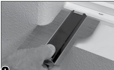
**6** Use a contour gauge to copy the radius of the bull nose.
