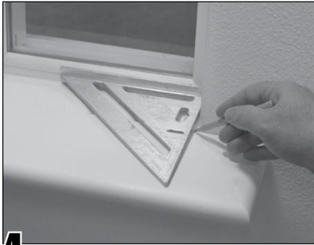
**4** Place a small square against the jamb of the window opening and mark the left and right sides of the sill.
