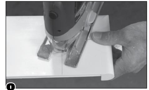
**8** Using a jigsaw, cut the curve. Continue with step 8 of the **Basic Installation Instructions**.
