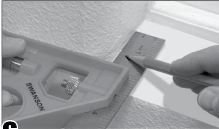
**6** Hold a combination square to the bull nose corner as shown. Locate the tangent point of the corner radius. Measure the distance.
