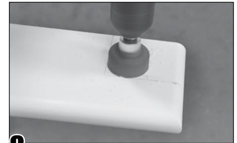
**8** Using the proper size hole saw bit, drill holes in the sill at the center points you marked.
