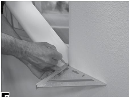
**5** Insert sill into the window opening at an angle with the back of the sill butt up against the window frame. With a square against the face of the wall, mark the depth of the window opening on the sill.
