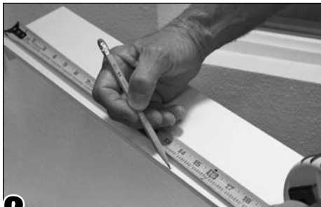
2 Measure and mark the center on the back of the sill.
