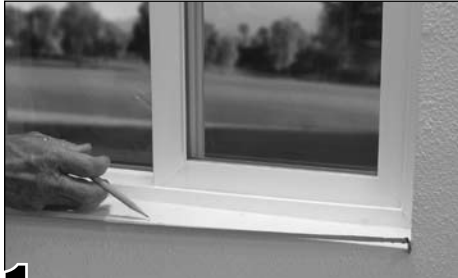
1 Measure and mark the center of the window.
