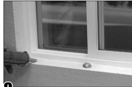
8 On the sill area, apply 1-inch balls of polyurethane construction adhesive three inches from each end and six inches apart.
