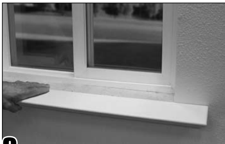
3 Align the center of the sill with the center of the window.
