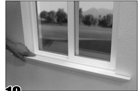
10 Insert the sill at a slight angle and making contact with the window then pivot the sill down in place.
